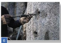
Use 34 mm ø (1") water pipe and put on tie bar
