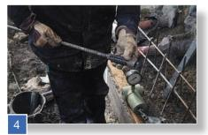
Screw the anchor onto the tie bar. Greasing the anchor facilitates the movement of the expandable jaws.
