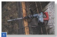
The hole needs to be round and smooth. The use of diamond tipped hollow core drill bits are recommended as they will cut through reinforcement without any problems. The drill should be properly guided by the use of a drill stand with a vacuum foot or a movable drill carriage.
