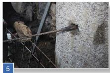
Insert anchor with tie bar into the drill hole and push it all the way to the bottom of the hole.
