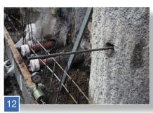
If the tie bar is required for fixing shuttering, insert it into the hole until it touches the back of the hole. This is important since the anchor will slip 10-20mm during the application of the test load (see 10) until the anchor reaches its final safe position. This will prevent the anchor from being loosened should it be accidentally knocked when positioning the formwork shutter.
