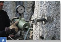
Position the hydraulic press onto the tie bar.
