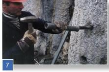
Hammer strokes on the pipe enable the expandable jaws to expend and to press their jaws into the concrete.
