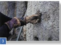
The drill hole has to be cleaned from dust. Because of possible dust remaining in the hole, the anchors always have to be inserted in a way that the expandable jaws are in an horizontal position.
