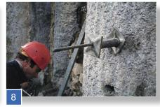
Take away the pipe, put a washer plate, a tube and a second washer plate on the tie bar.
