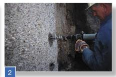
If only a few drill holes are required it may be more economic to use a standard drill with a carbide tipped drill bit. The main disadvantages of this are: the high effort required by the user for holding and pressing, the high amount of dust created, non circular holes and the number unfinished holes due to clashes with reinforcement.
